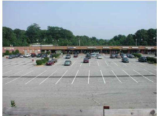
Excess Pavement Increases Runoff
