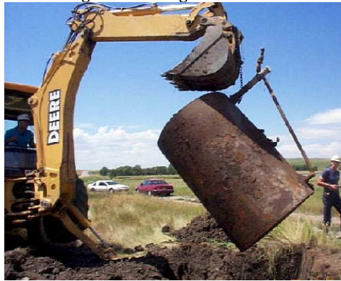
Underground Storage Tank Removal
